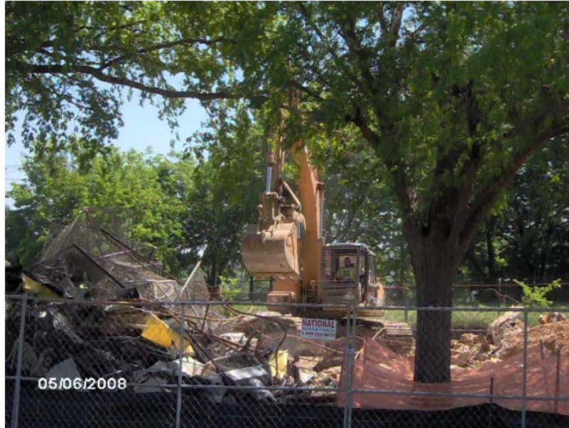
TUXEDO COURT DEMOLITION OF DAYCARE
