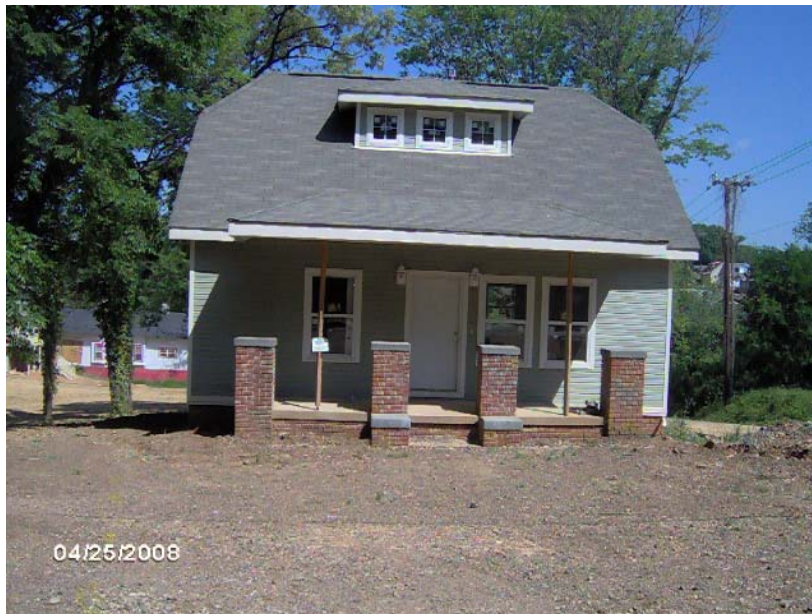
TUXEDO COURT LOT 13 IN FOUNTAIN HEIGHTS CONSTRUCTION PROGRESS
