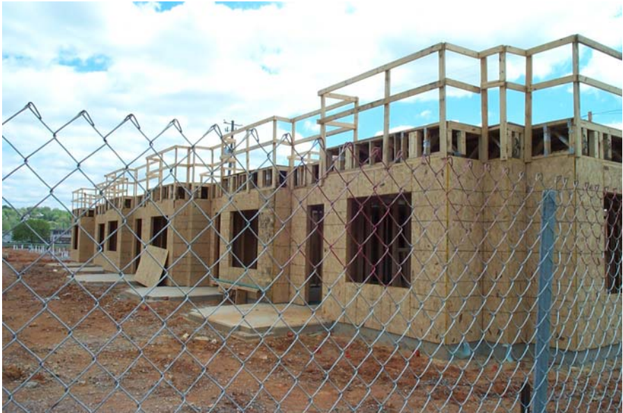
TUXEDO COURT RENTAL UNITS CONSTRUCTION PROGRESS BLOCK 2 LOOKING SOUTHEAST
