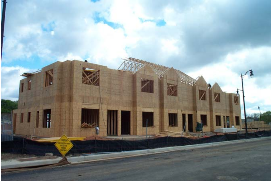
TUXEDO COURT RENTAL UNITS CONSTRUCTION PROGRESS BLOCK 6 LOOKING SOUTHWEST
