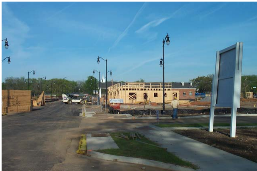
TUXEDO COURT RENTAL UNITS CONSTRUCTION PROGRESS BLOCK 2 LOOKING WEST
