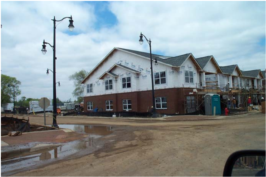
TUXEDO COURT RENTAL UNITS CONSTRUCTION PROGRESS BLOCK 6 LOOKING NORTHWEST
