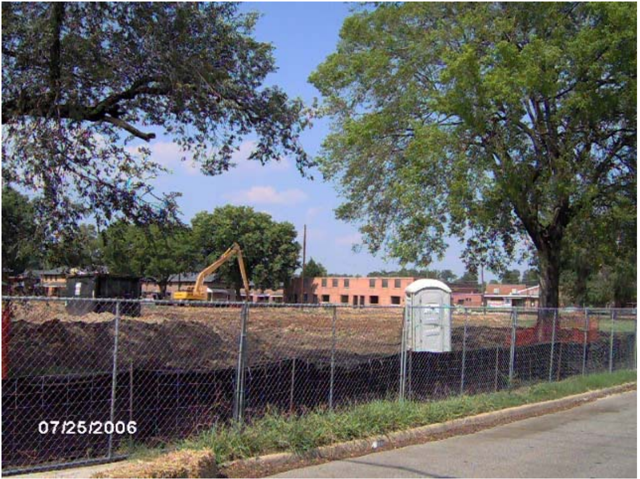
TUXEDO COURT DEMOLITION SERVICES ON BLOCK 6 AT TUXEDO COURT
