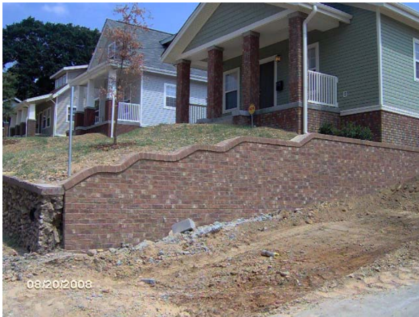
TUXEDO COURT LOT 21 IN FOUNTAIN HEIGHTS RETAINING WALL CONSTRUCTION
