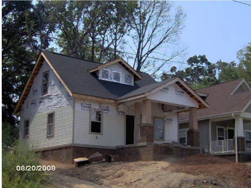
TUXEDO COURT LOT 17 IN FOUNTAIN HEIGHTS CONSTRUCTION PROGRESS
