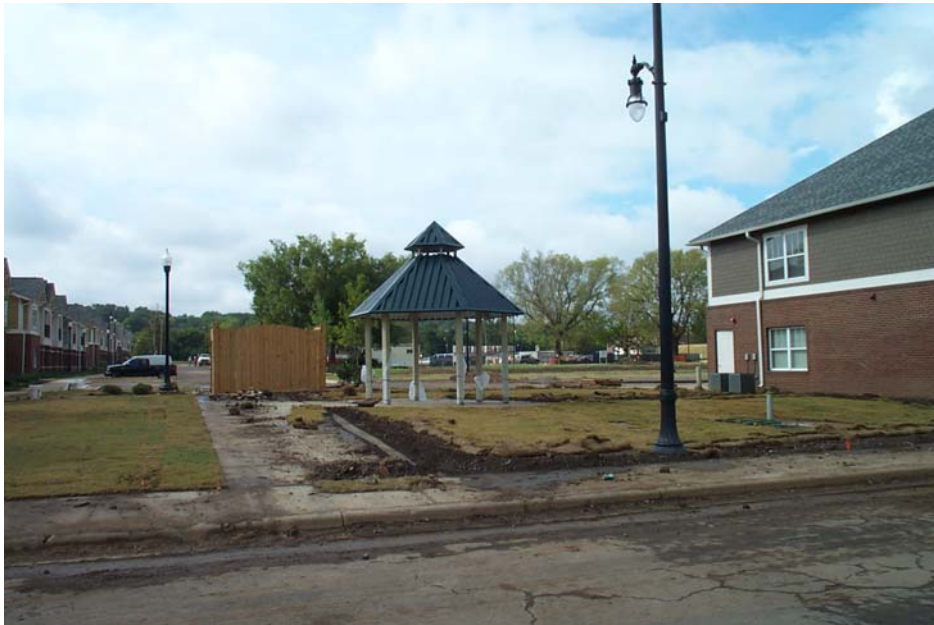
TUXEDO COURT RENTAL UNITS CONSTRUCTION PROGRESS GAZEBO – BLOCK 6
