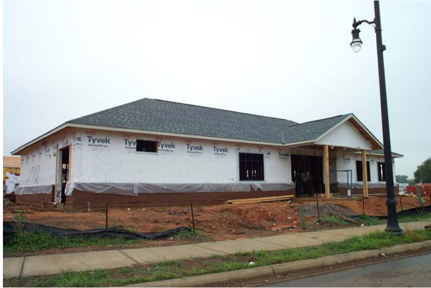
TUXEDO COURT RENTAL UNITS CONSTRUCTION PROGRESS COMMUNITY BUILDING - BLOCK 4
