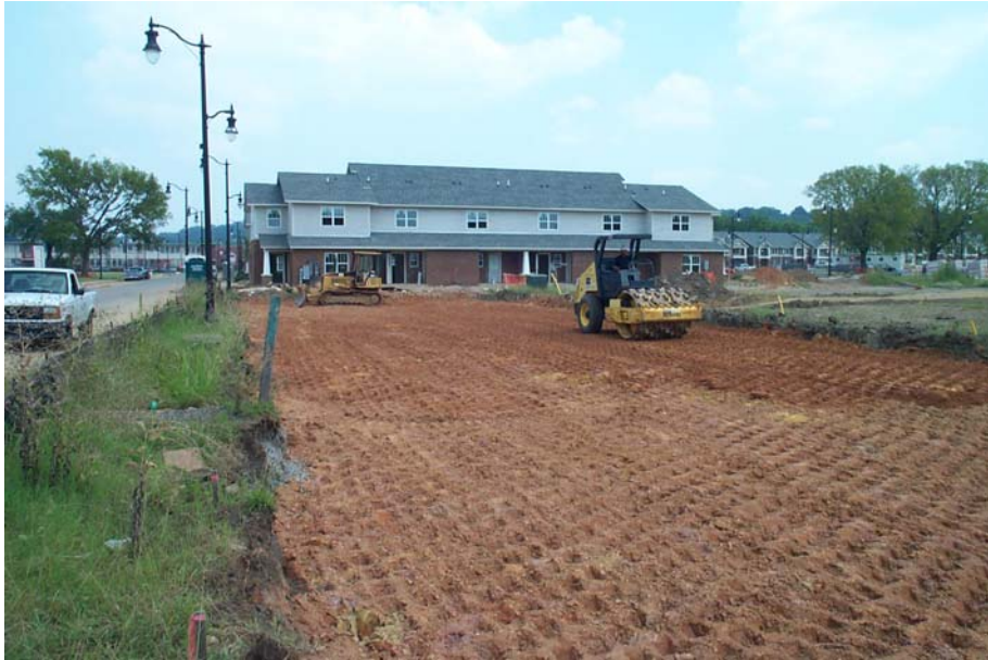
TUXEDO COURT RENTAL UNITS CONSTRUCTION PROGRESS COMPACTION PROCESSES – BLOCK 5
