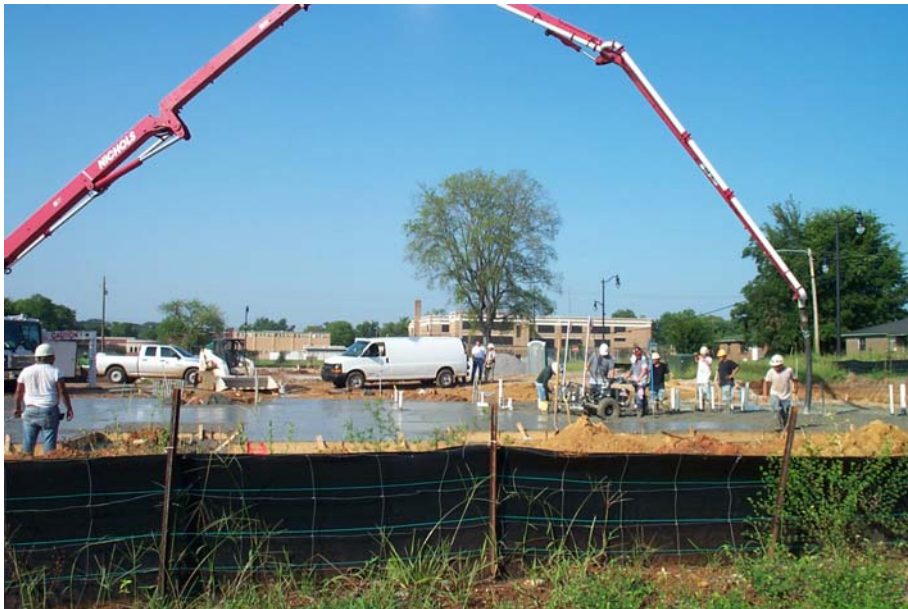
TUXEDO COURT RENTAL UNITS CONSTRUCTION PROGRESS FOUNDATION CONSTRUCTION - BLOCK 7
