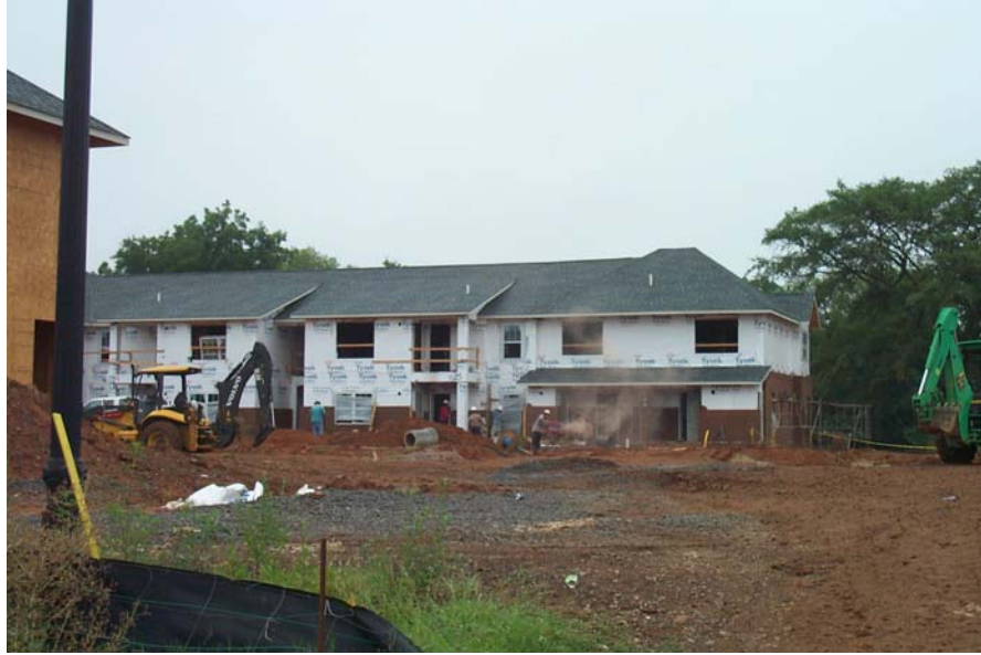
TUXEDO COURT RENTAL UNITS CONSTRUCTION PROGRESS BLOCK 2
