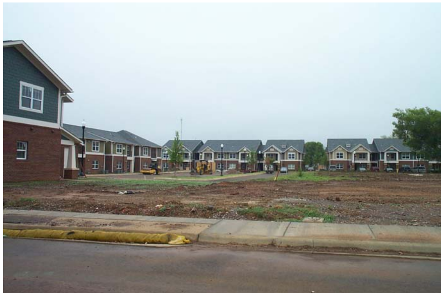
TUXEDO COURT RENTAL UNITS CONSTRUCTION PROGRESS BLOCK 6 – LOOKING EAST
