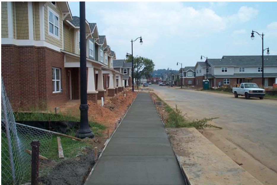
TUXEDO COURT RENTAL UNITS CONSTRUCTION PROGRESS SIDEWALK CONSTRUCTION – BLOCK 2
