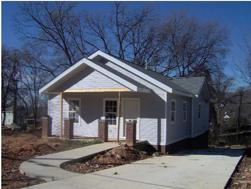
TUXEDO COURT LOT 16 IN FOUNTAIN HEIGHTS CONSTRUCTION PROGRESS
