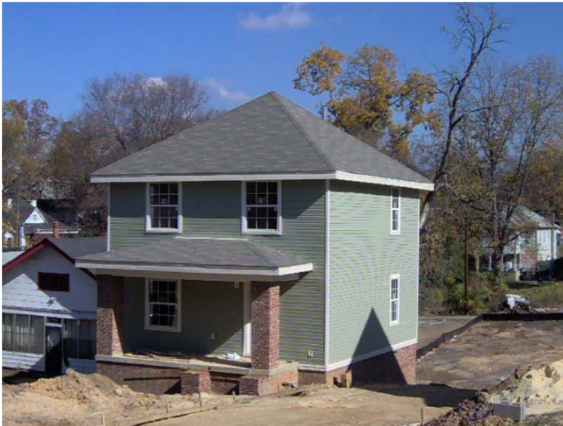
TUXEDO COURT LOT 9 IN FOUNTAIN HEIGHTS PROGRESS
