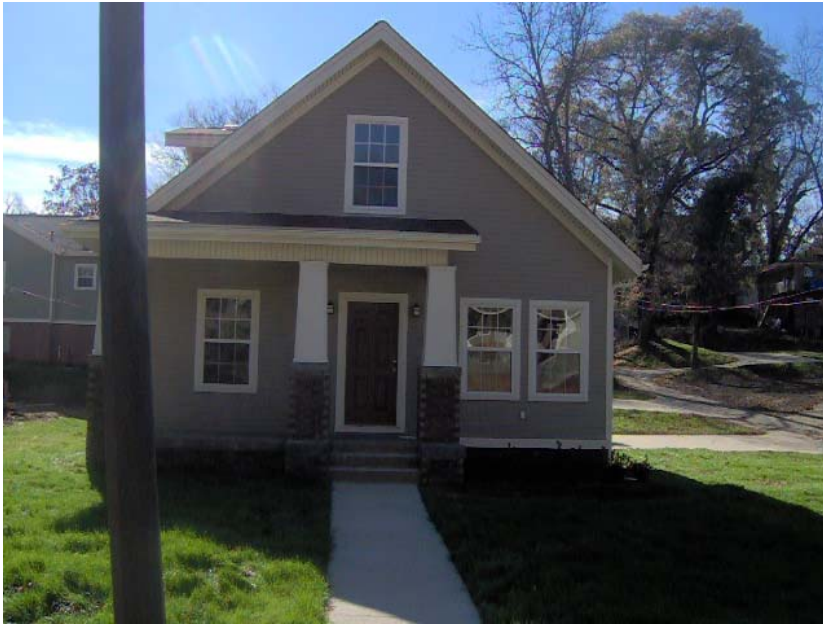
TUXEDO COURT LOT 4 IN FOUNTAIN HEIGHTS PROGRESS
