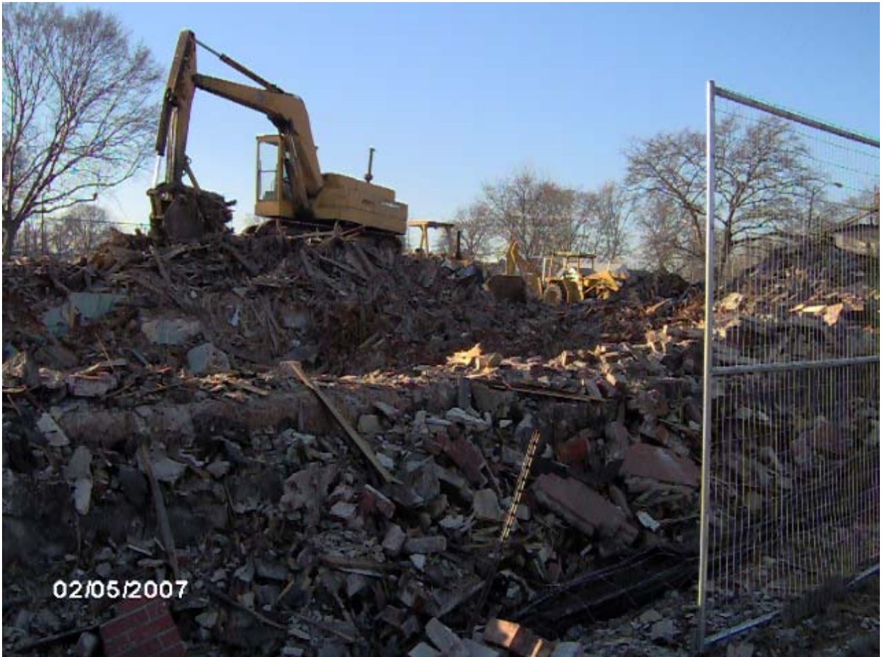
TUXEDO COURT DEMOLITION OF PROPERTY AT 1436 20 TH PLACE ENSLEY ON FEBRUARY 5, 2007
