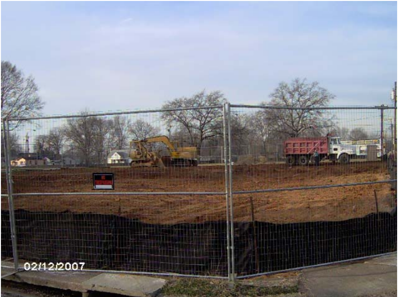
TUXEDO COURT DEMOLITION OF PROPERTY AT 1436 20 TH PLACE ENSLEY ON FEBRUARY 12, 2007
