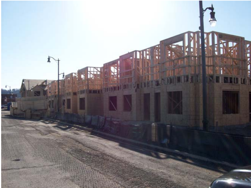
TUXEDO COURT RENTAL UNITS CONSTRUCTION PROGRESS BLOCK 6 LOOKING EAST
