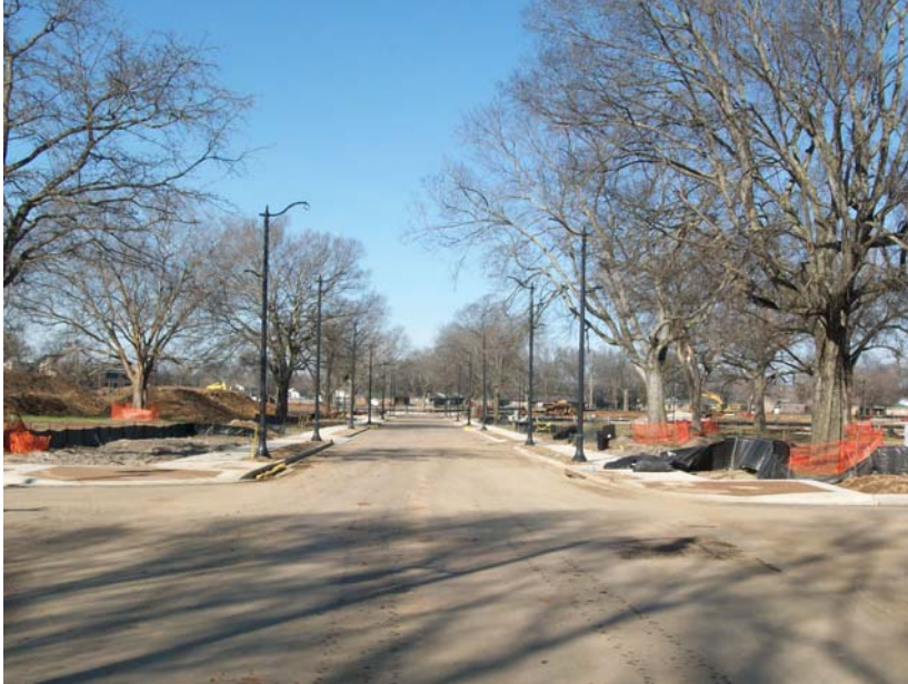
TUXEDO COURT INFRASTRUCTURE CONSTRUCTION PROGRESS NEW STREETS AND LIGHTING
