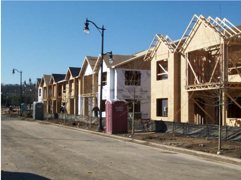
TUXEDO COURT RENTAL UNITS CONSTRUCTION PROGRESS BLOCK 6 – LOOKING SOUTH
