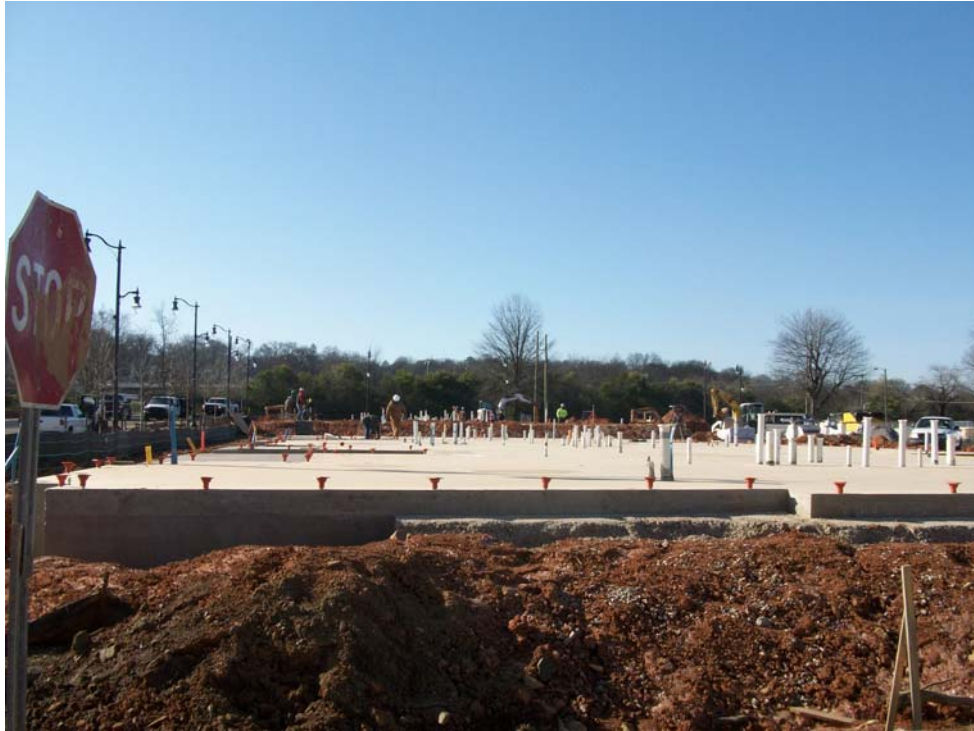
TUXEDO COURT RENTAL UNITS CONSTRUCTION PROGRESS FOUNDATIONS ON BLOCK 10 – LOOKING SOUTH
