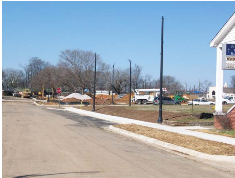
TUXEDO COURT INFRASTRUCTURE CONSTRUCTION PROGRESS NEW STREETS, CURBS, AND LIGHTING
