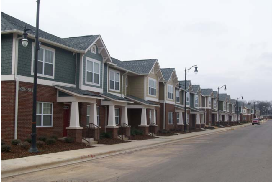
TUXEDO COURT RENTAL UNITS CONSTRUCTION PROGRESS BLOCK 5
