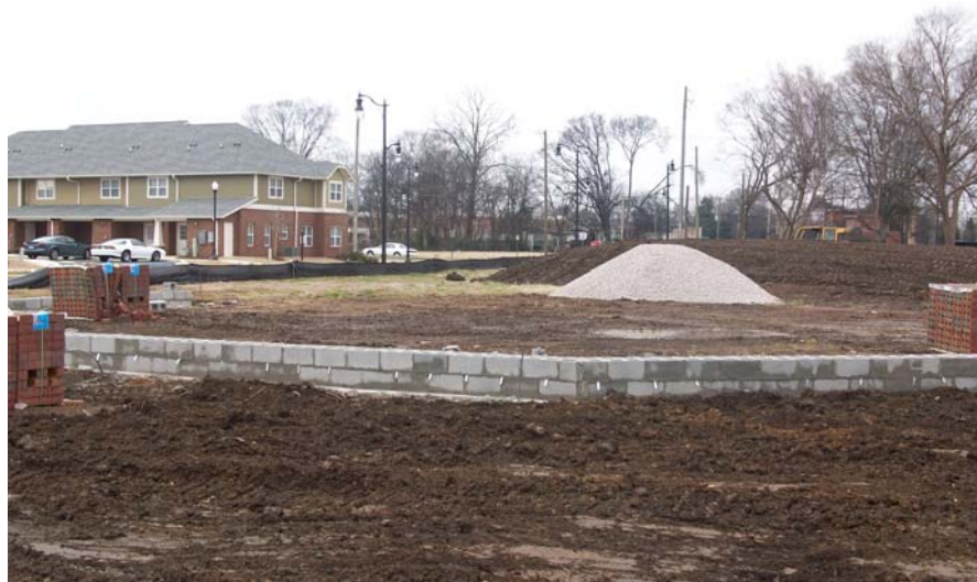
TUXEDO COURT GATEWAY PARK CONSTRUCTION PROGRESS BLOCK 3
