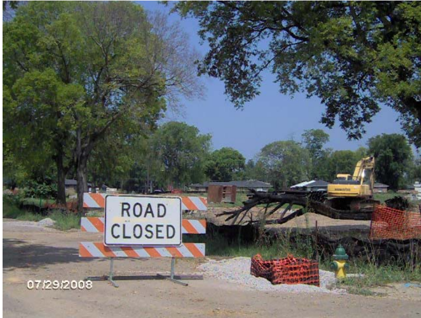
TUXEDO COURT INFRASTRUCTURE CONSTRUCTION PROGRESS
