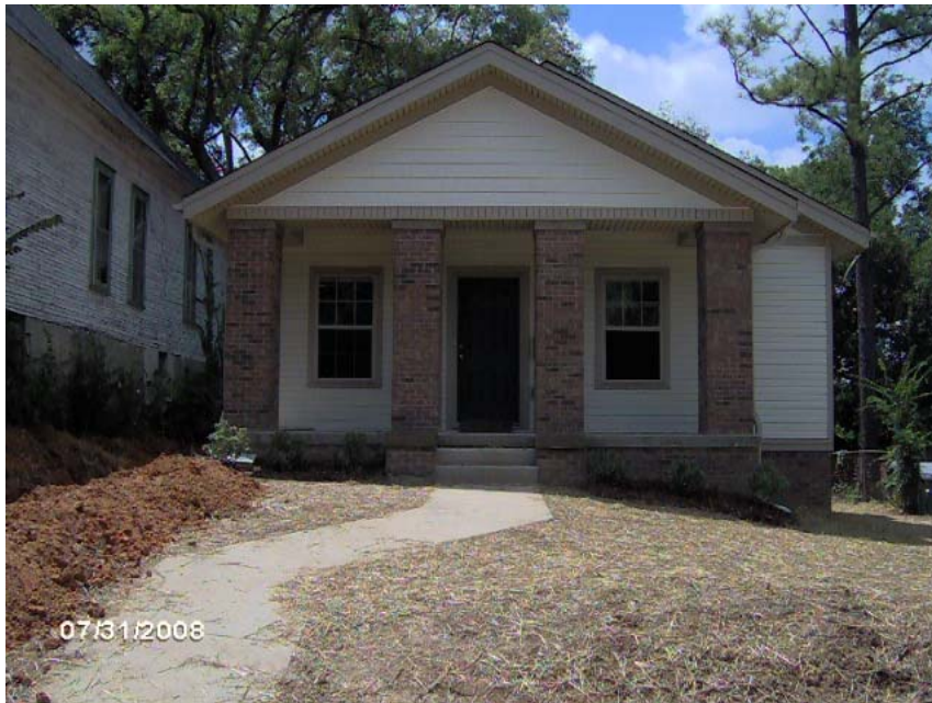
TUXEDO COURT LOT 27 IN FOUNTAIN HEIGHTS ON JULY 31ST CONSTRUCTION PROGRES
