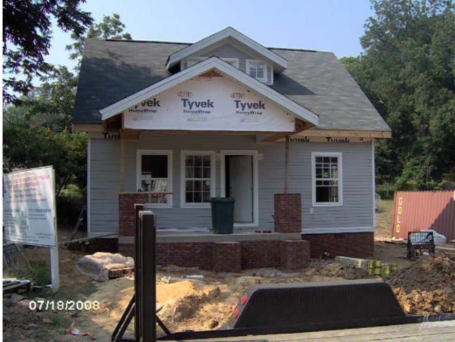
TUXEDO COURT LOT 5 IN FOUNTAIN HEIGHTS CONSTRUCTION PROGRESS
