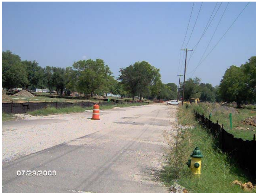
TUXEDO COURT INFRASTRUCTURE CONSTRUCTION PROGRESS
