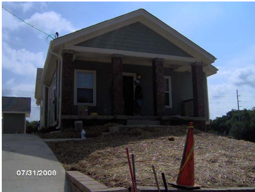
TUXEDO COURT LOT 21 IN FOUNTAIN HEIGHTS ON JULY 31 CONSTRUCTION PROGRESS
