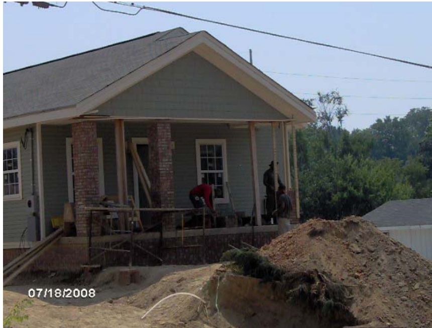
TUXEDO COURT LOT 21 IN FOUNTAIN HEIGHTS ON JULY 18TH CONSTRUCTION PROGRESS
