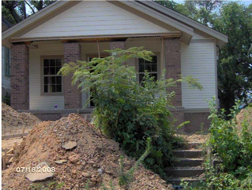
TUXEDO COURT LOT 27 IN FOUNTAIN HEIGHTS ON JULY 18TH CONSTRUCTION PROGRESS
