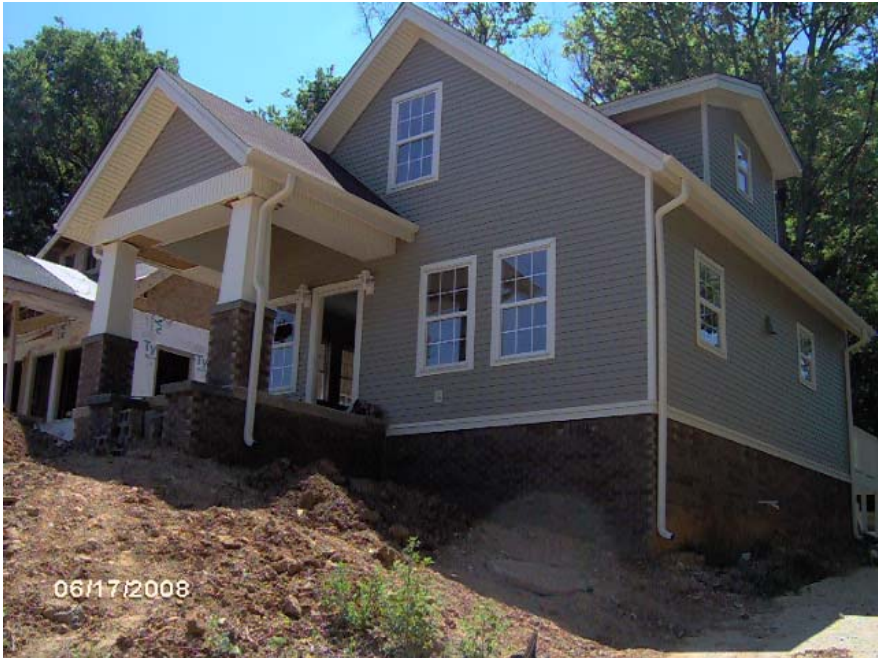
TUXEDO COURT LOT 18 IN FOUNTAIN HEIGHTS CONSTRUCTION PROGRESS
