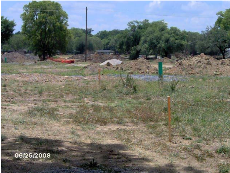
TUXEDO COURT INFRASTRUCTURE CONSTRUCTION CONSTRUCTION STAKING
