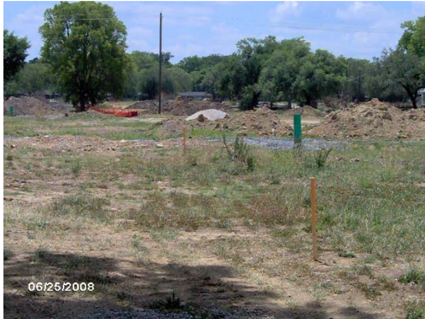
TUXEDO COURT INFRASTRUCTURE CONSTRUCTION CONSTRUCTION STAKING
