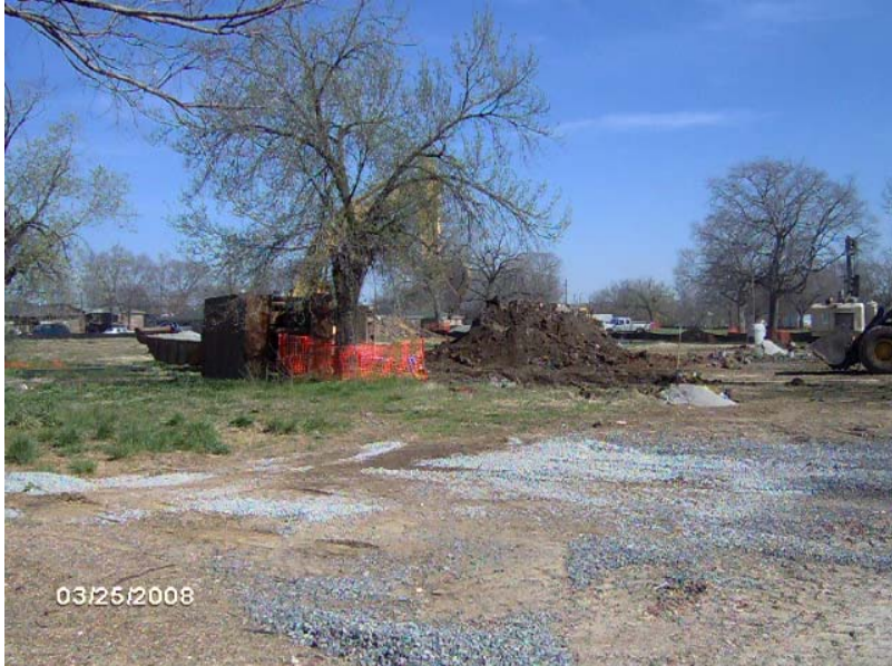
TUXEDO COURT INFRASTRUCTURE CONSTRUCTION SANITARY SEWER
