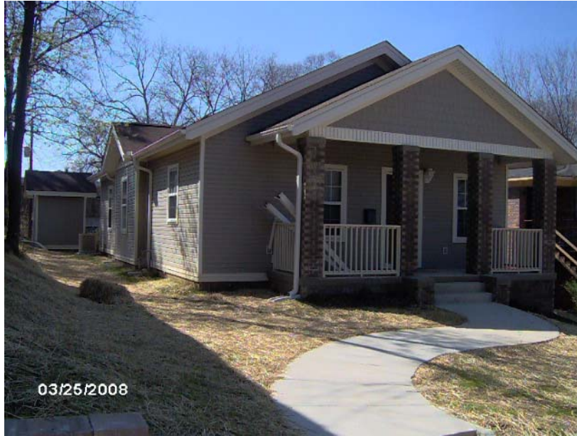
TUXEDO COURT LOT 8 IN FOUNTAIN HEIGHTS FINISHING TOUCHES
