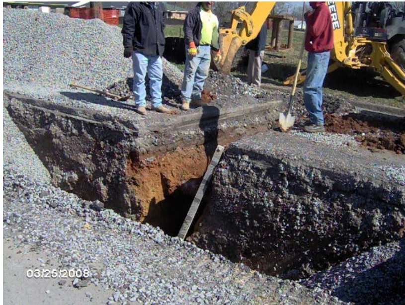
TUXEDO COURT INFRASTRUCTURE CONSTRUCTION TRENCHING
