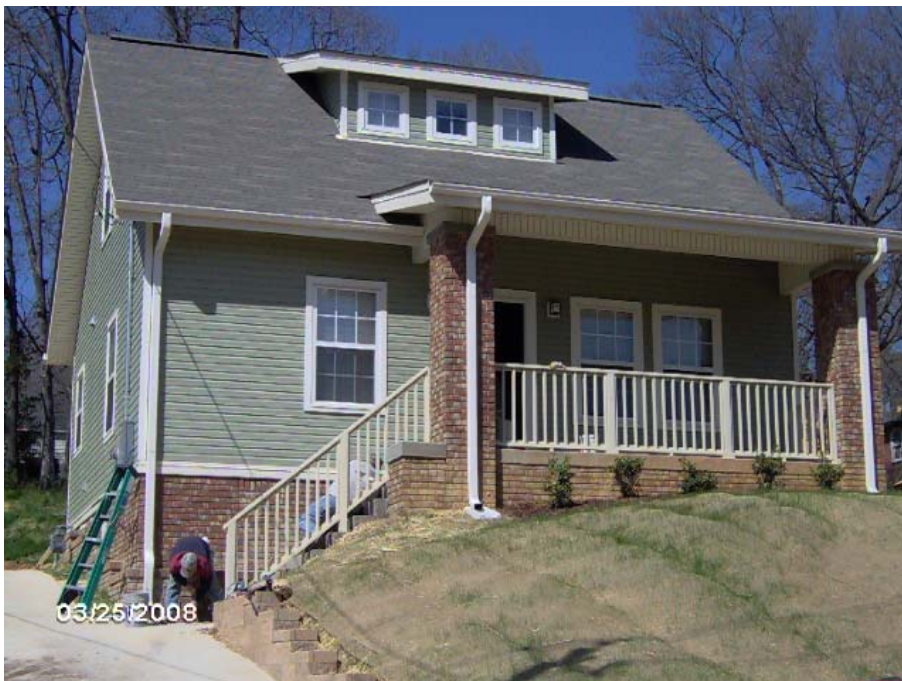
TUXEDO COURT LOT 41 IN FOUNTAIN HEIGHTS CONSTRUCTION PROGRESS
