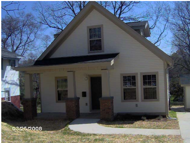
TUXEDO COURT LOT 25 IN FOUNTAIN HEIGHTS CONSTRUCTION PROGRESS
