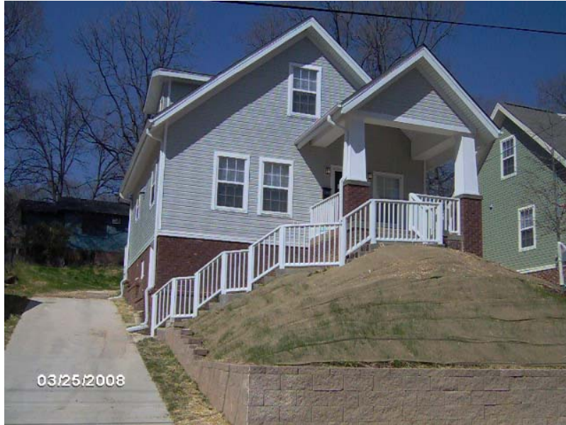
TUXEDO COURT LOT 40 IN FOUNTAIN HEIGHTS FINISHING TOUCHES
