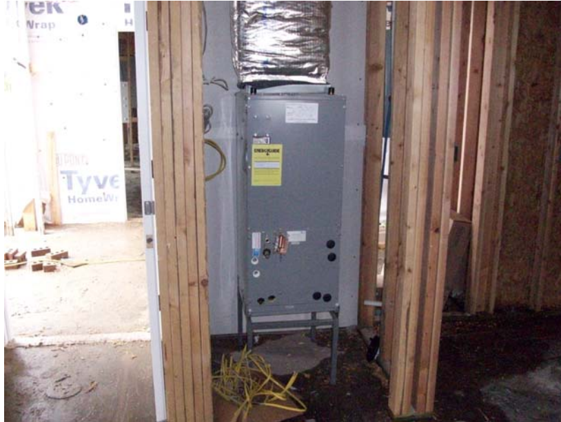
TUXEDO COURT RENTAL UNITS CONSTRUCTION PROGRESS HVAC INSTALLATION
