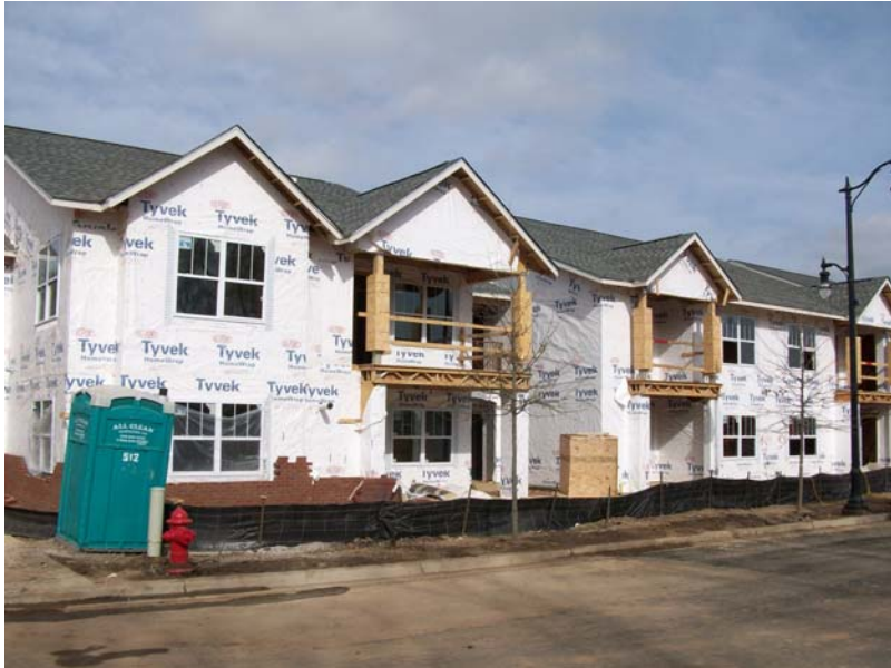
TUXEDO COURT RENTAL UNITS CONSTRUCTION PROGRESS BLOCK 6 LOOKING NORTHWEST
