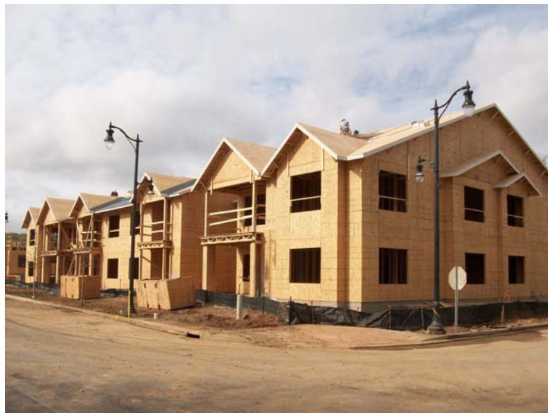
TUXEDO COURT RENTAL UNITS CONSTRUCTION PROGRESS BLOCK 6 LOOKING SOUTHEAST
