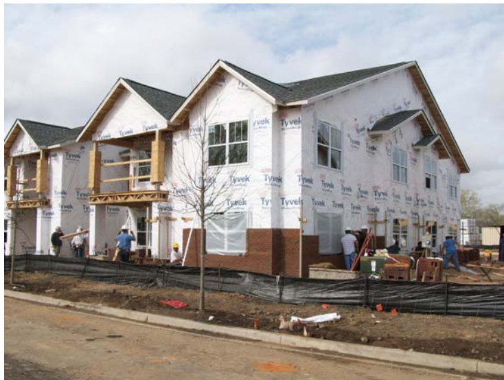
TUXEDO COURT RENTAL UNITS CONSTRUCTION PROGRESS BLOCK 6 LOOKING SOUTHWEST
