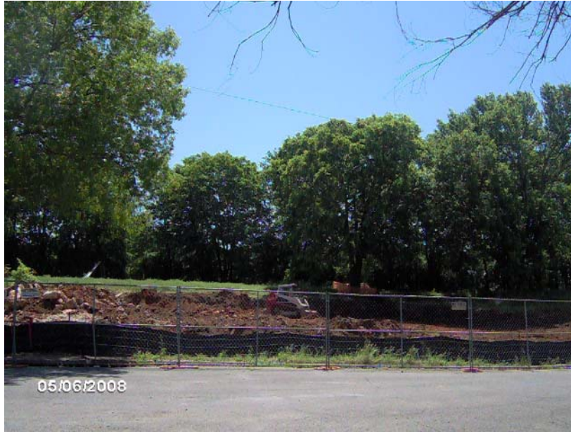
TUXEDO COURT ON SITE DEMOLITION
