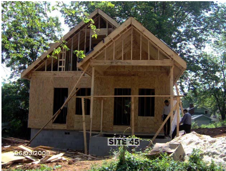
TUXEDO COURT LOT 45 IN FOUNTAIN HEIGHTS CONSTRUCTION PROGRESS
