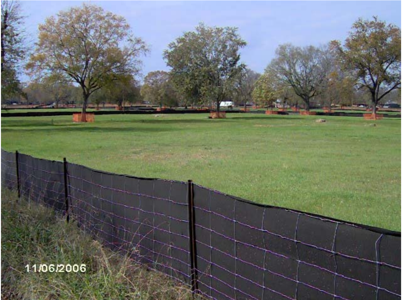
TUXEDO COURT DEMOLITION SERVICES Block 5 (looking northwest from 21 st Street Ensley)
