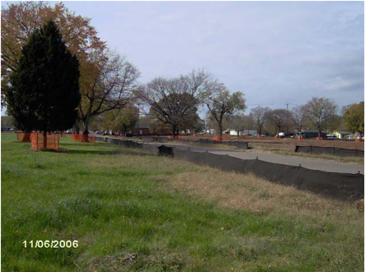
TUXEDO COURT DEMOLITION SERVICES Blocks 2 and 5 (looking northwest along 20 th Place)
