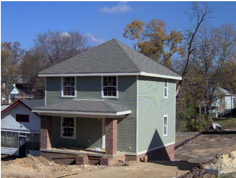
TUXEDO COURT LOT 9 IN FOUNTAIN HEIGHTS PROGRESS
