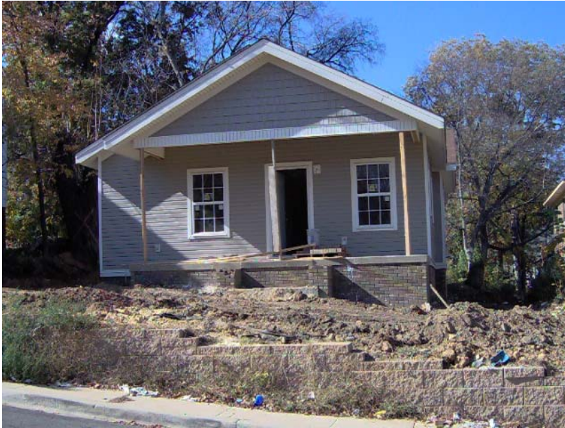
TUXEDO COURT LOT 8 IN FOUNTAIN HEIGHTS PROGRESS
