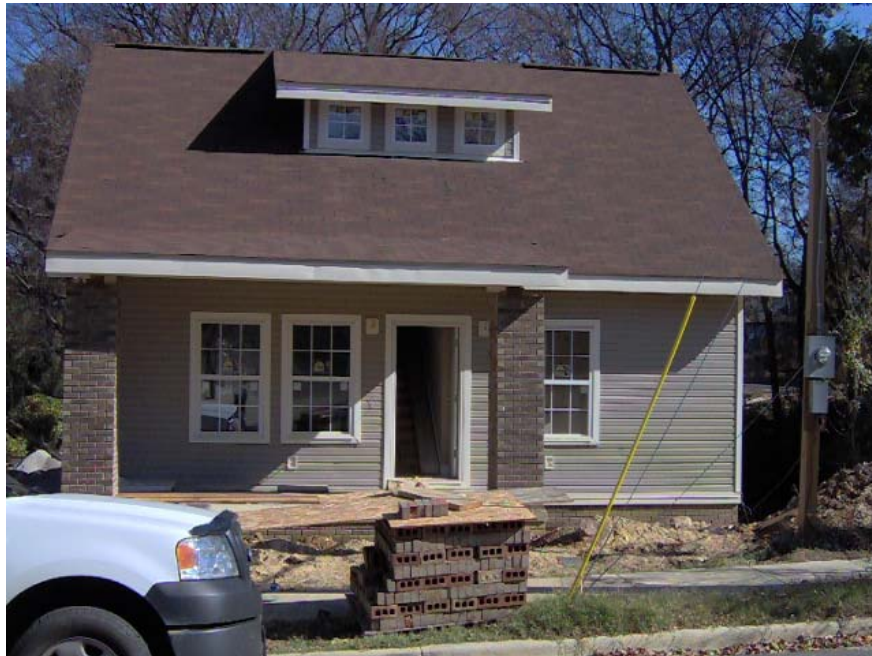
TUXEDO COURT LOT 12 IN FOUNTAIN HEIGHTS CONSTRUCTION PROGRESS
