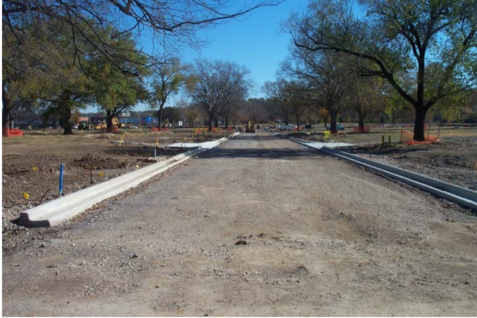
TUXEDO COURT INFRASTRUCTURE CONSTRUCTION PROGRESS CURB AND GUTTER INSTALLATION
