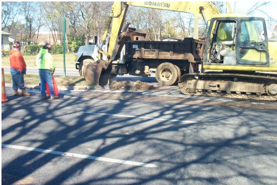
TUXEDO COURT INFRASTRUCTURE CONSTRUCTION PROGRESS CLOSING THE 20 TH STREET MEDIAN
