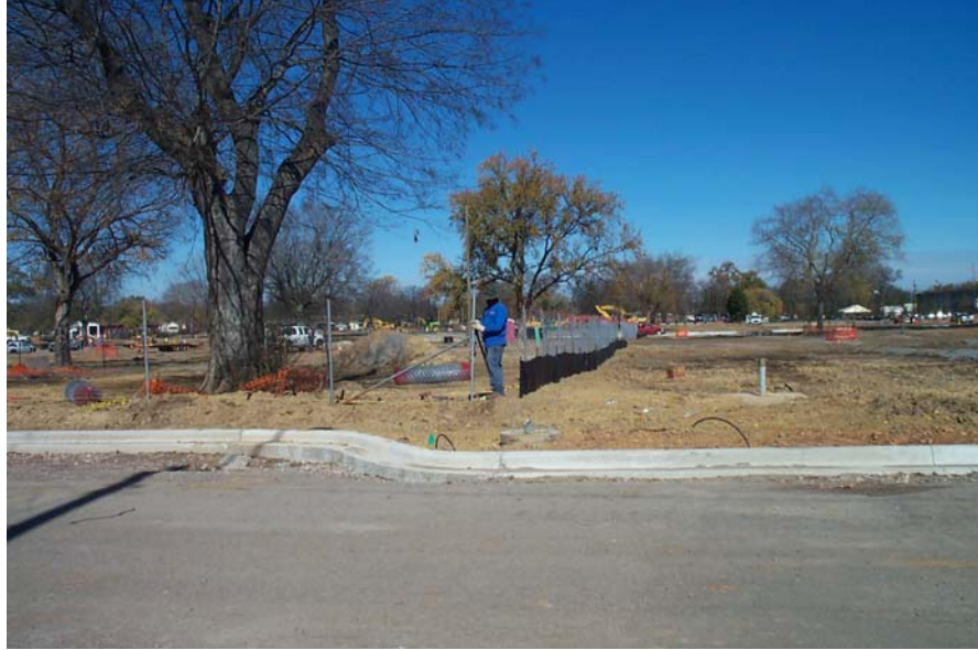
TUXEDO COURT RENTAL UNITS CONSTRUCTION PROGRESS SILT FENCE INSTALLATION
