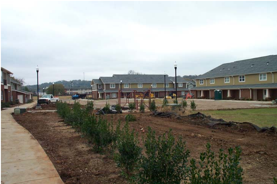
TUXEDO COURT RENTAL UNITS CONSTRUCTION PROGRESS BLOCK 2 - LANDSCAPING SERVICES
