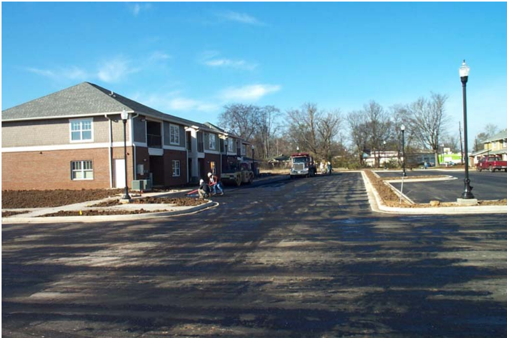
TUXEDO COURT RENTAL UNITS CONSTRUCTION PROGRESS BLOCK 2 – PARKING LOT PAVING
