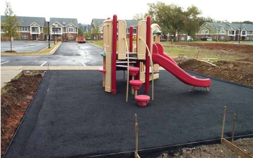
TUXEDO COURT RENTAL UNITS CONSTRUCTION PROGRESS BLOCK 6 – PLAYGROUND CONSTRUCTION
