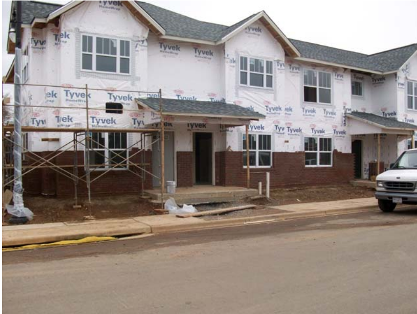
TUXEDO COURT RENTAL UNITS CONSTRUCTION PROGRESS BLOCK 5 – ONGOING CONSTRUCTION
