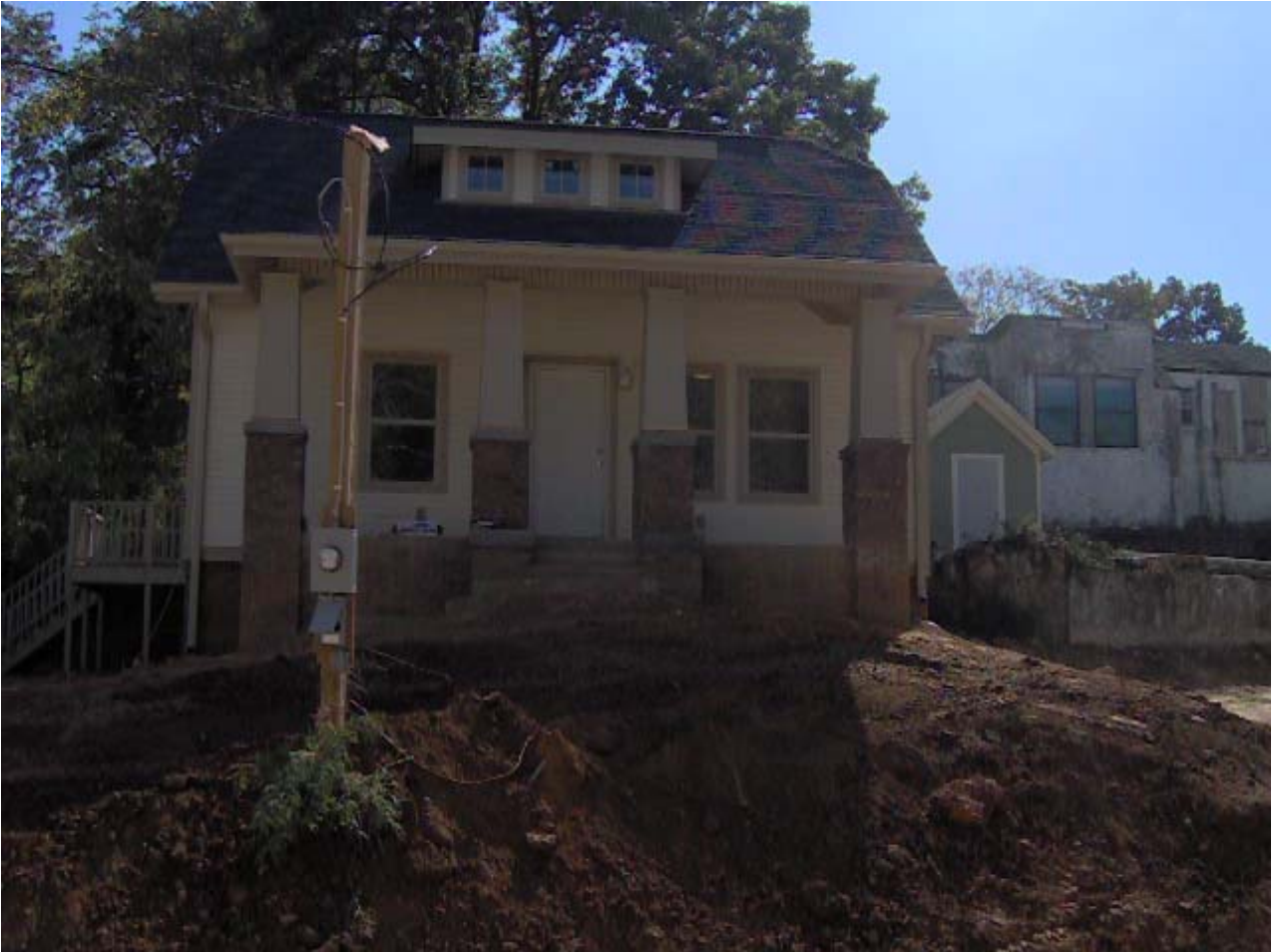
TUXEDO COURT LOT 3 ALONG 15 TH AVENUE NORTH IN FOUNTAIN HEIGHTS PROGRESS
