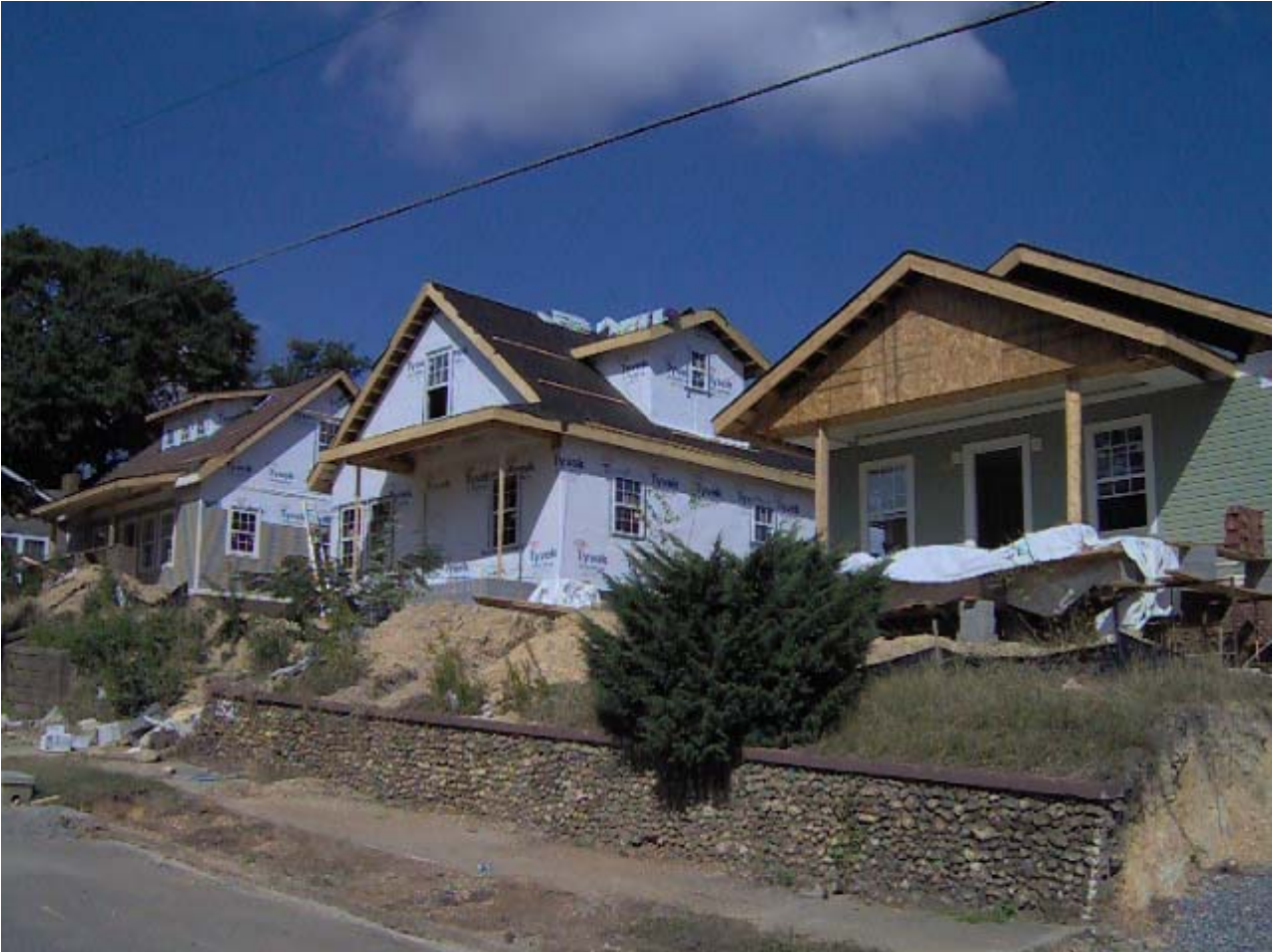
TUXEDO COURT LOTS 21, 22, AND 23 IN FOUNTAIN HEIGHTS CONSTRUCTION PROGRESS
