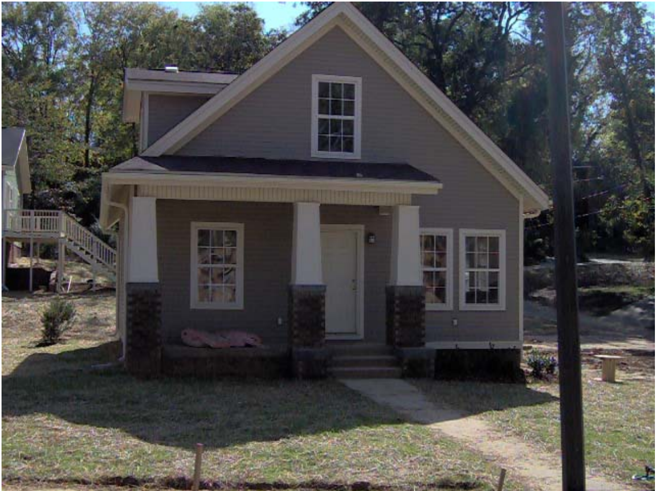
TUXEDO COURT LOT 4 IN FOUNTAIN HEIGHTS GRADING PROGRESS - LOOKING LIKE HOME
