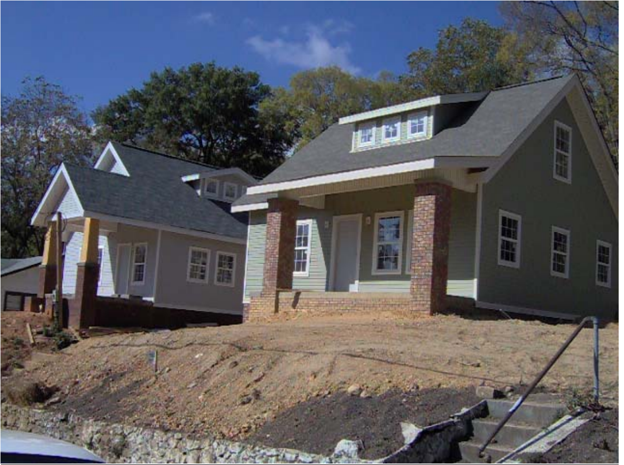
TUXEDO COURT LOTS 40 AND 41 IN FOUNTAIN HEIGHTS GRADING PROGRESS
