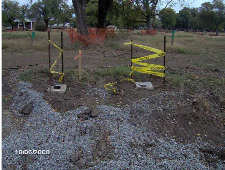
TUXEDO COURT INFRASTRUCTURE CONSTRUCTION PROGRESS INSTALLATION OF METERS
