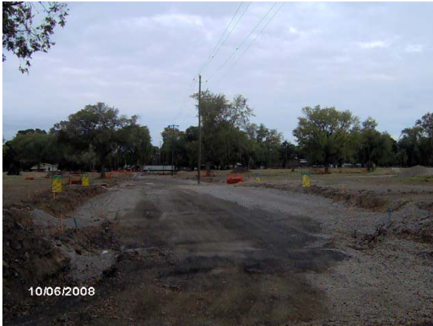
TUXEDO COURT INFRASTRUCTURE CONSTRUCTION PROGRESS INSTALLATION OF A NEW ROAD
