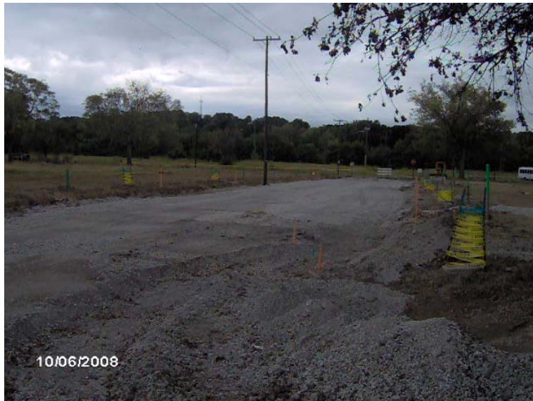
TUXEDO COURT INFRASTRUCTURE CONSTRUCTION PROGRESS WATER LINE INSTALLATION
