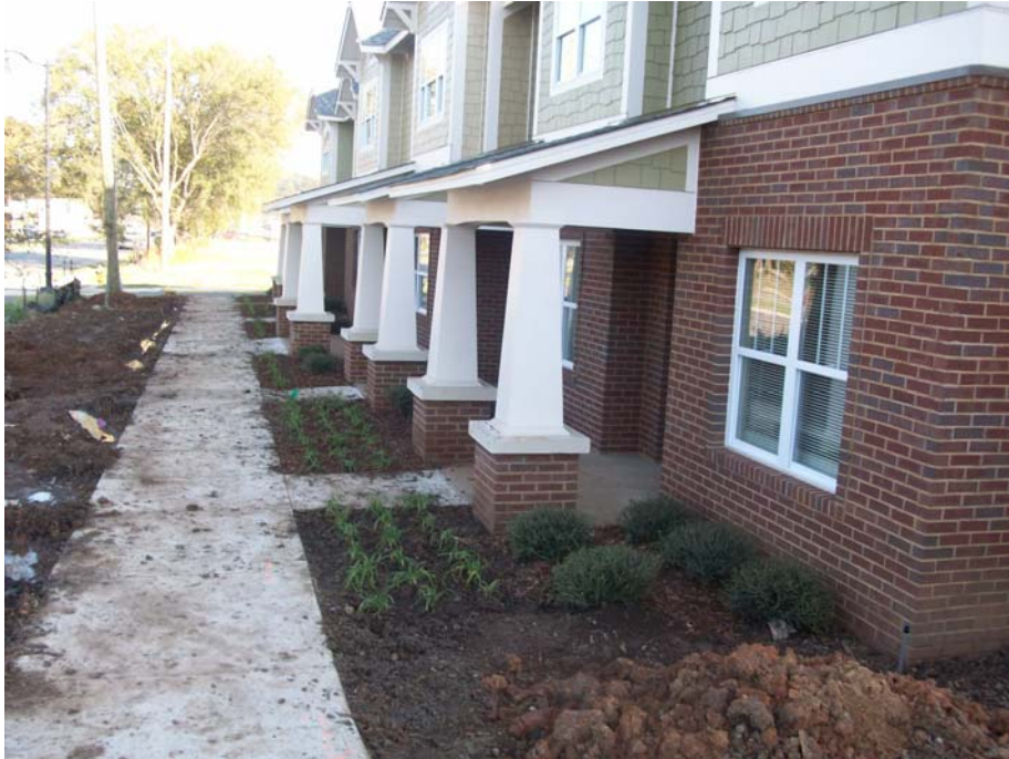
TUXEDO COURT RENTAL UNITS CONSTRUCTION PROGRESS LANDSCAPING SERVICES
