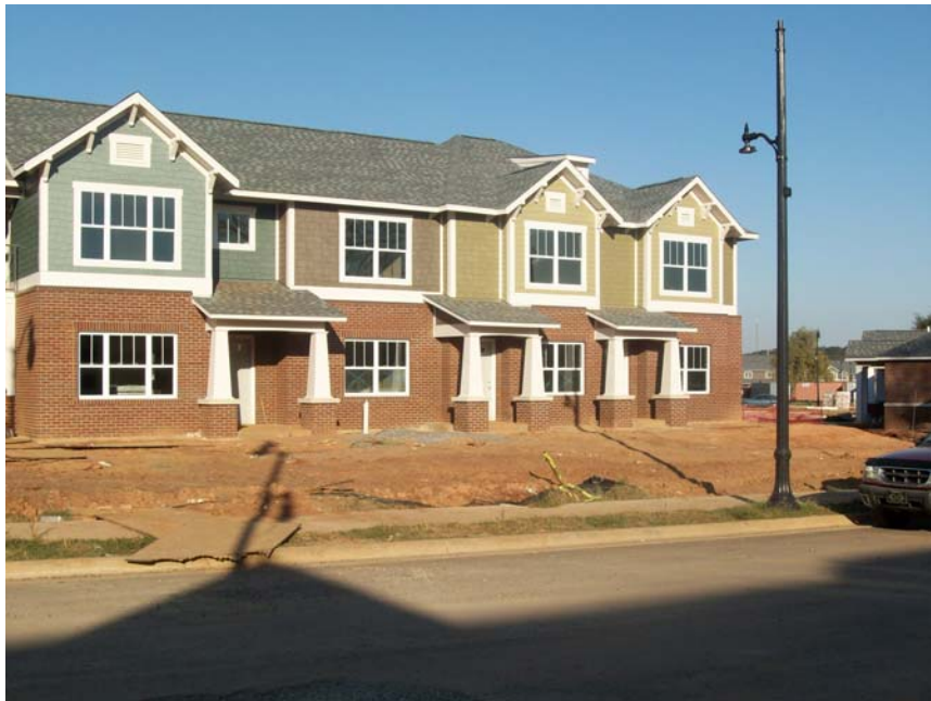
TUXEDO COURT RENTAL UNITS CONSTRUCTION PROGRESS BLOCK 7
