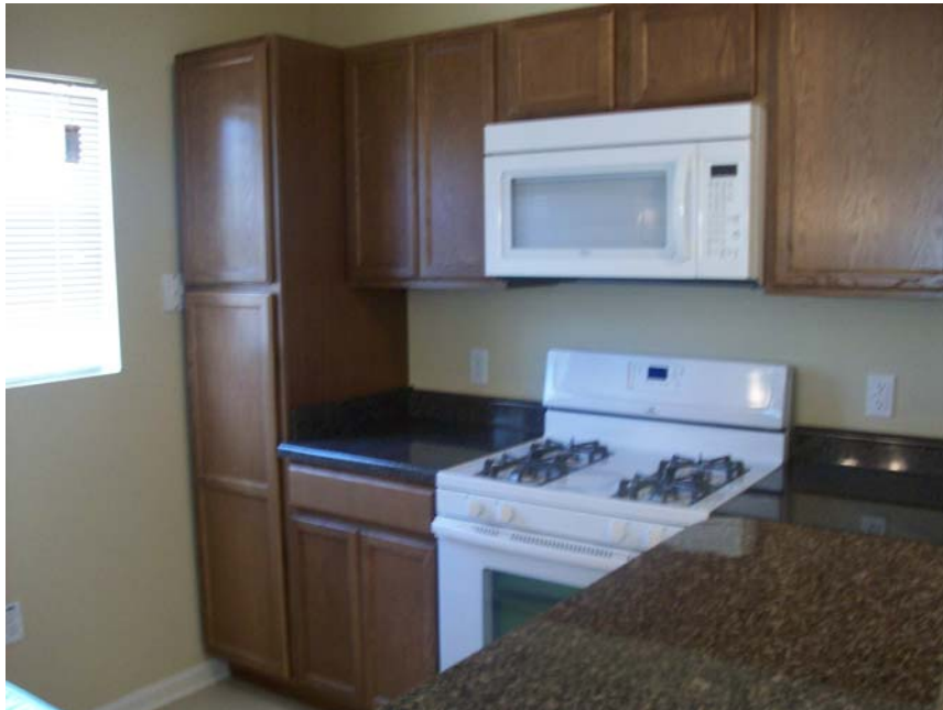
TUXEDO COURT RENTAL UNITS CONSTRUCTION PROGRESS INTERIORS
