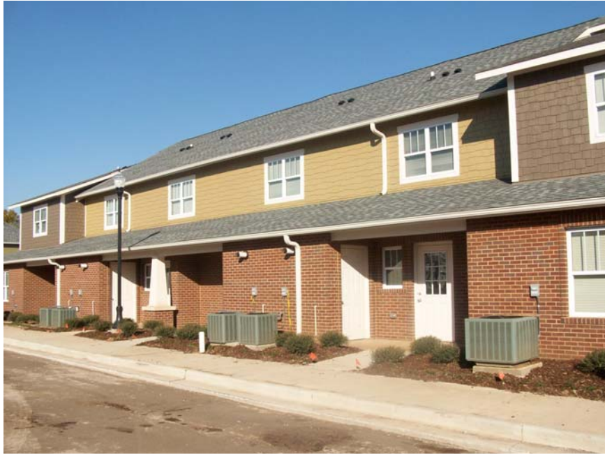
TUXEDO COURT RENTAL UNITS CONSTRUCTION PROGRESS BLOCK 6 – PARKING LOT VIEW
