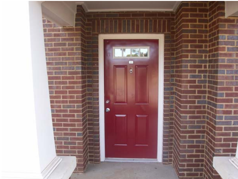
TUXEDO COURT RENTAL UNITS CONSTRUCTION PROGRESS LOOKING LIKE HOME
