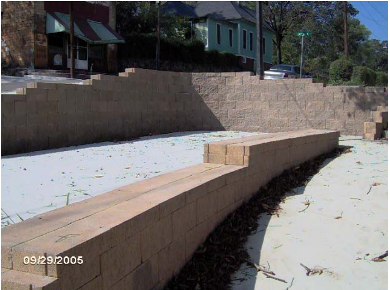
TUXEDO COURT CONSTRUCTION PROGRESS AT THE NORTHERN TRIANGLE IN THE FOUNTAIN HEIGHTS NEIGHBORHOOD
