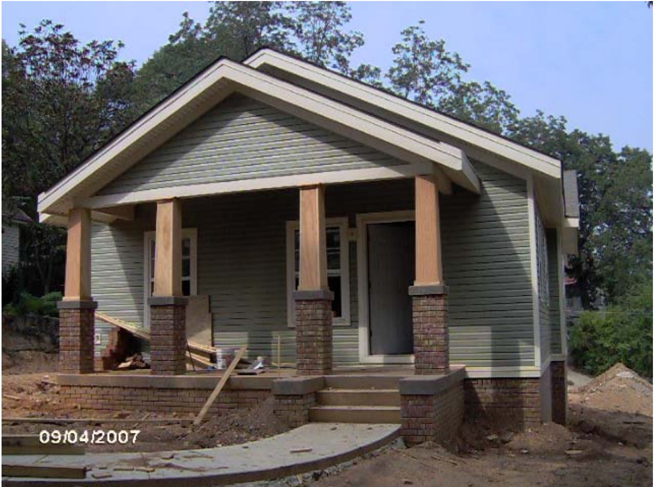
TUXEDO COURT LOT 6 ALONG 16 TH STREET NORTH IN FOUNTAIN HEIGHTS PROGRESS
