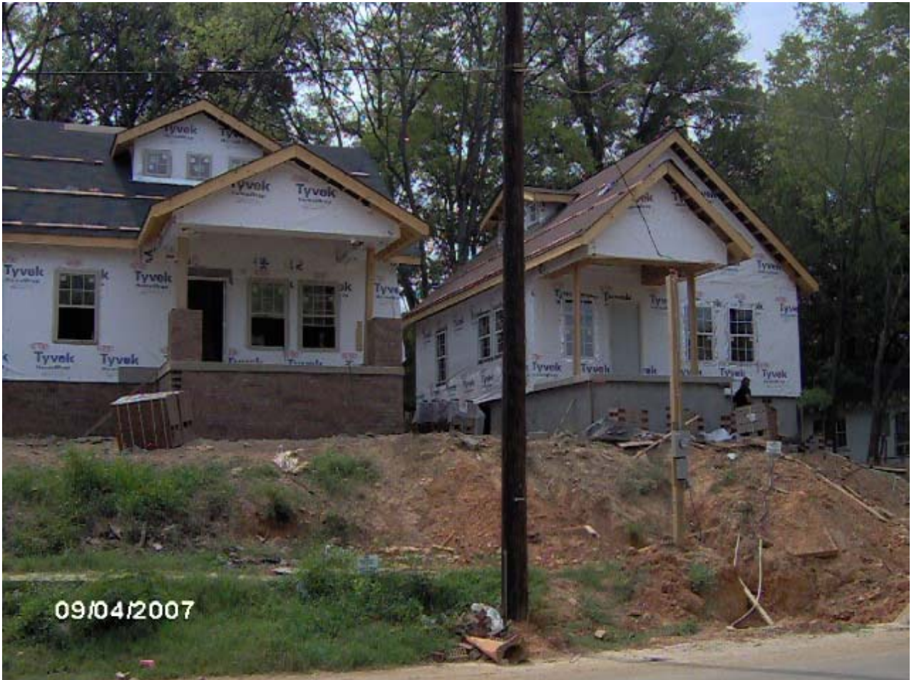
TUXEDO COURT LOTS 17 AND 18 IN FOUNTAIN HEIGHTS CONSTRUCTION PROGRESS
