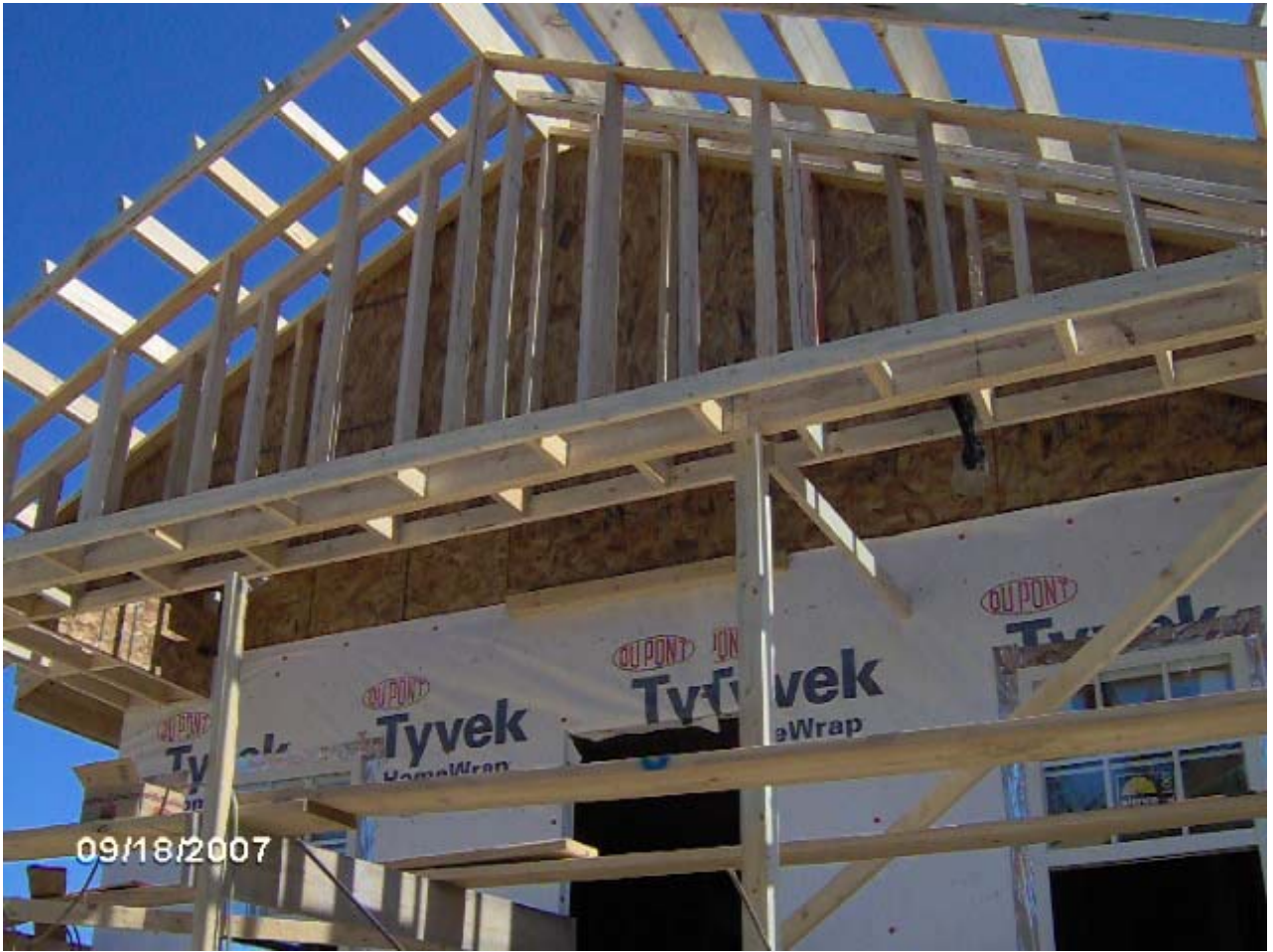
TUXEDO COURT LOT 21 IN FOUNTAIN HEIGHTS ROUGH CARPENTRY PROGRESS
