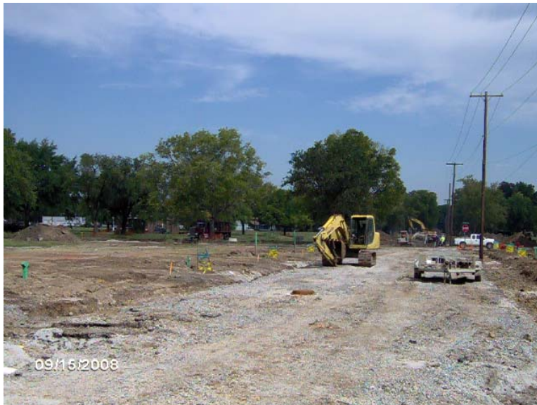
TUXEDO COURT INFRASTRUCTURE CONSTRUCTION PROGRESS
