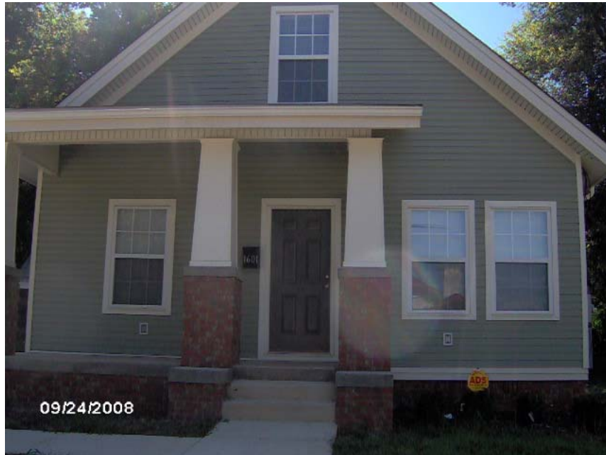
TUXEDO COURT LOT 20 IN FOUNTAIN HEIGHTS CONSTRUCTION PROGRESS
