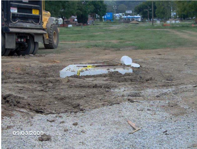
TUXEDO COURT INFRASTRUCTURE CONSTRUCTION PROGRESS
