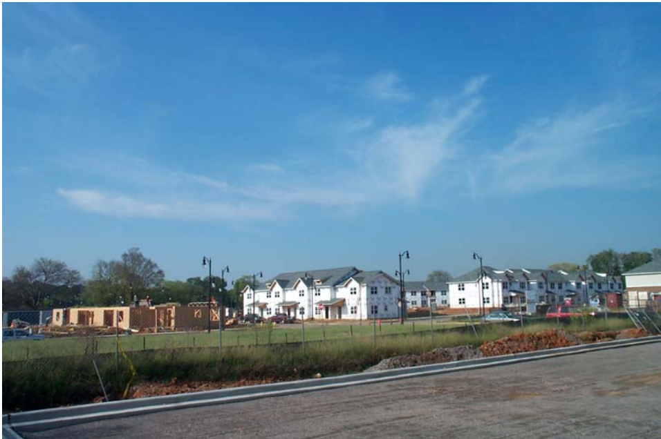
TUXEDO COURT RENTAL UNITS CONSTRUCTION PROGRESS SITE OVERVIEW
