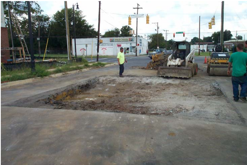
TUXEDO COURT RENTAL UNITS CONSTRUCTION PROGRESS INFRASTRUCTURE IMPROVEMENTS
