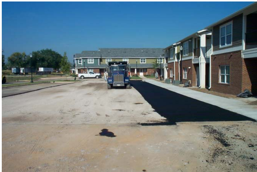
TUXEDO COURT RENTAL UNITS CONSTRUCTION PROGRESS BLOCK 6 – PARKING LOT PAVING
