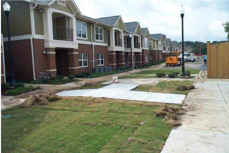
TUXEDO COURT RENTAL UNITS CONSTRUCTION PROGRESS LANDSCAPING SERVICES – BLOCK 6
