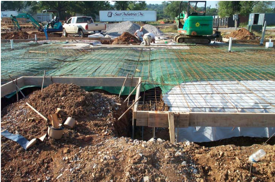
TUXEDO COURT RENTAL UNITS CONSTRUCTION PROGRESS FOUNDATIONS
