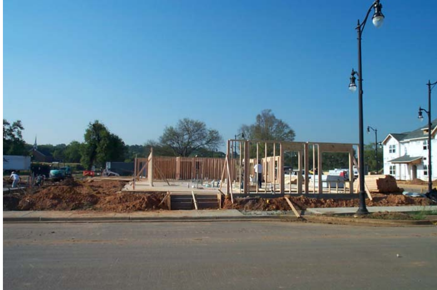
TUXEDO COURT RENTAL UNITS CONSTRUCTION PROGRESS BLOCK 7
