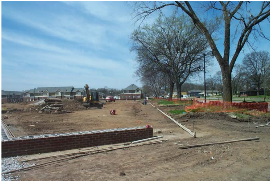
TUXEDO COURT CONSTRUCTION PROGRESS GATEWAY PARK CONSTRUCTION - BLOCK 3
